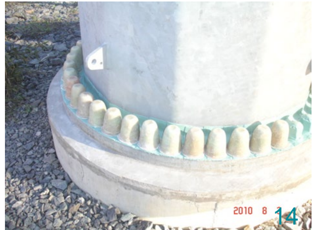
Wrappingband EZ can be painted with a topcoat.
