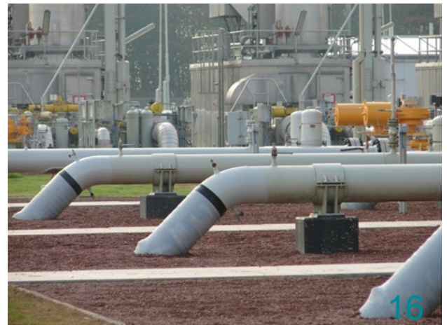
Paint the above ground part of the riser with a UV resistant topcoat to prevent discoloration of the Outerglass Shield XT.
