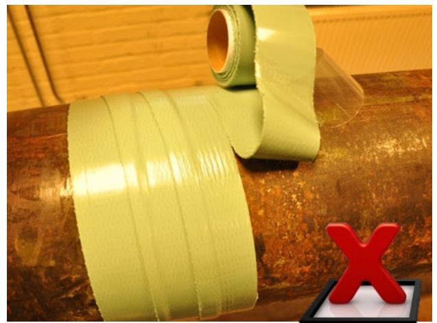
Minimum side by side overlap shall be 10mm. Use the indication line printed on the Wrappingband, present on all Wrappingband wider than 50mm.
