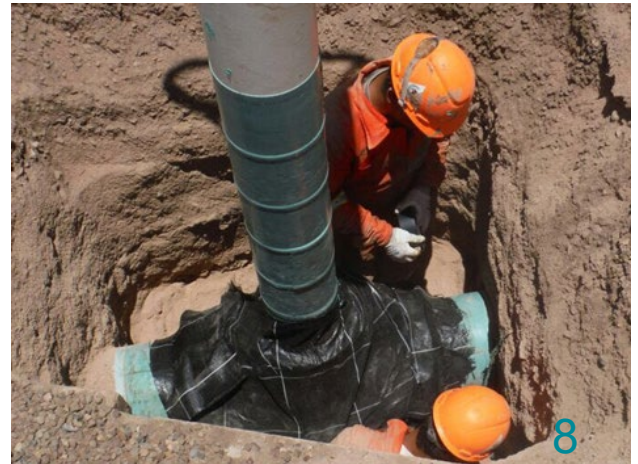
The Geotextile shall cover all the applied 4100 Putty.
