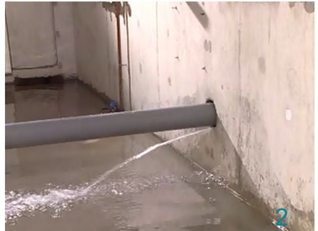
The sealing system can be applied while the duct is leaking.
