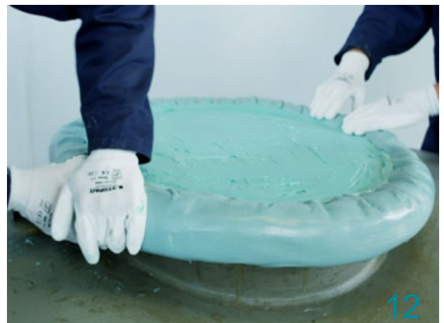
The Wrappingband will not adhere to the 4100 Putty. The width of the Wrappingband should be sufficient so that the bolts and nuts are covered.
