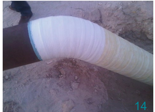
Paint the above ground part of the riser with a UV resistant topcoat to prevent discoloration of the Outerglass Shield XT.
