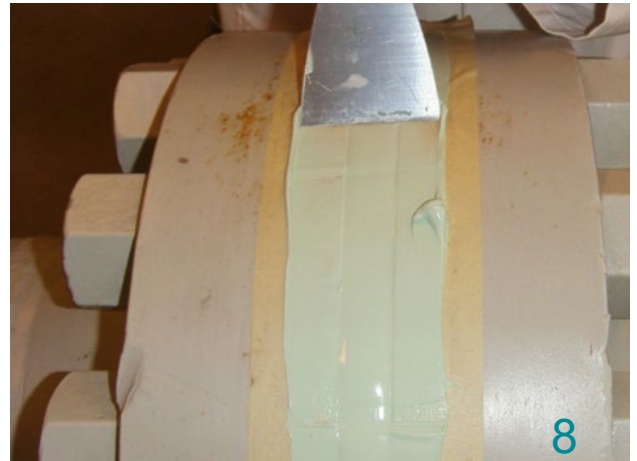
Prevent 4200 Filler from adhering to the surface of the flange.
