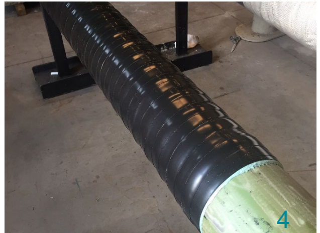
Outerwrap shall always be applied by means of spiral wrap with a minimum side-by-side overlap of 50%.
