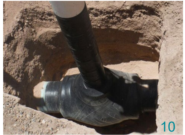
Apply Outerwrap by means of spiral wrap over the adjacent pipes with a minimum overlap of 50%. Apply with tension, avoid air inclusions and keep approx. 3-5mm of Wrappingband visible.
