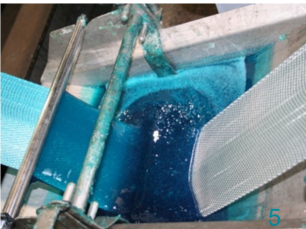
Mix the POWERCRETE parts A, B and C with the pigments as per the mixing ratios given in the PDS to ensure the best performance. Pour the mixed epoxy in the FAST GRE Wrapping Device.
