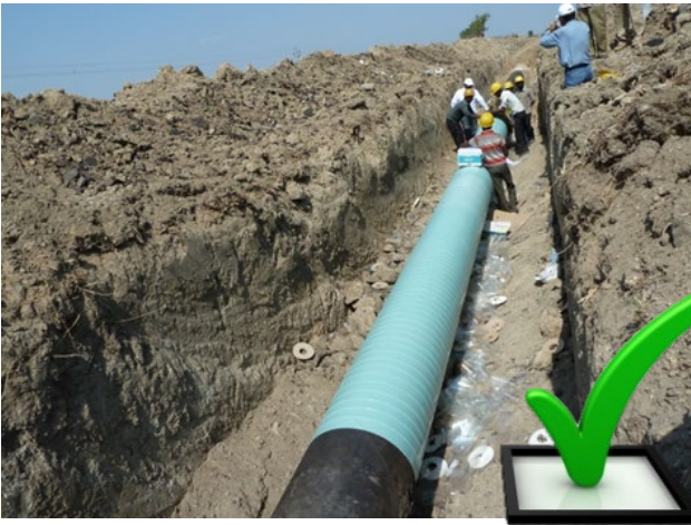
Start and end with a straight circumferential wrap.
