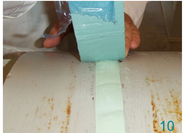
Wrappingband shall be applied without air entrapment. Fold the Wrappingband back into the Paste.
