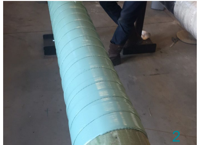
Wrappingband can be applied with straight wraps or by means of spiral wrap.
