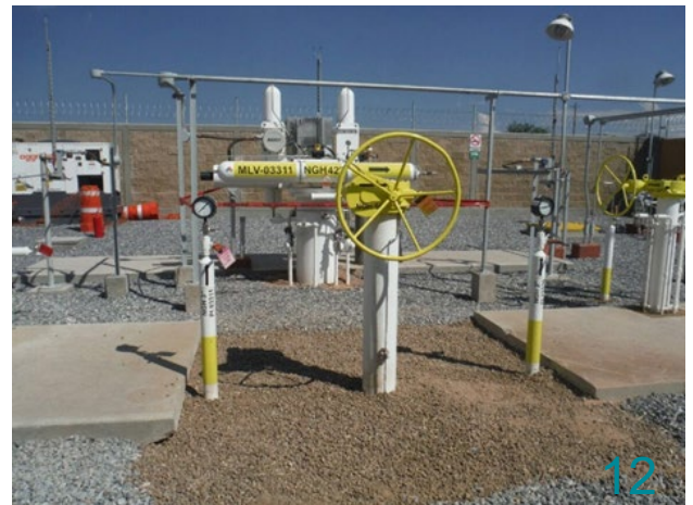
If the STOPAQ® system has to be applied in soil-to-air transition areas, additional layers of Outerglass Shield XT shall be applied at the transition area.
