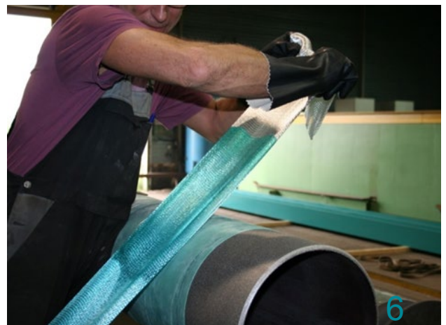
Pull the impregnated FAST GRE Fabric through the GRE Wrapping Device and place it on the FAST Basecoat GRE.
