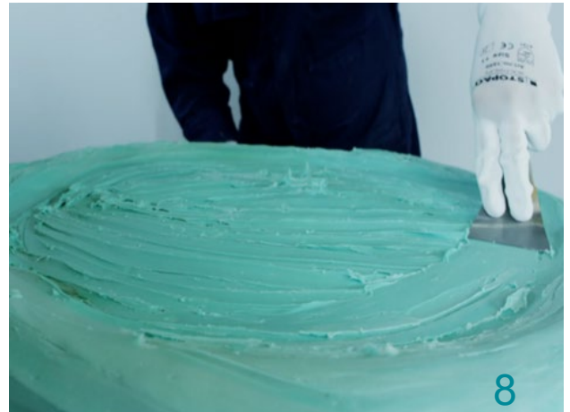
A putty knife can be used to smooth the surface of the 4100 Putty.
