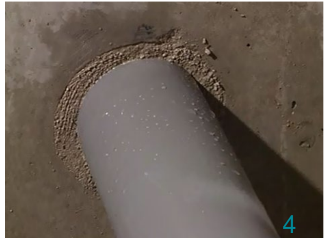
Mortar FR for ducts with Flame retardant properties Mortar WR for ducts with Water resistant properties
