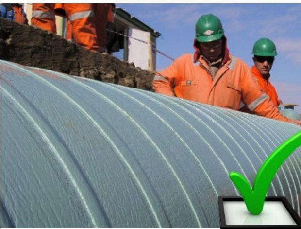
Minimum side by side overlap shall be 10mm. Use the indication line printed on the Wrappingband, present on all Wrappingband wider than 50mm.
