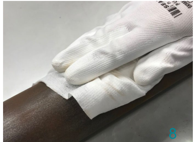
After folding the SFL® Cleaning Wipe the surface can be cleaned. Firmly rub the entire surface with the Wipe.
