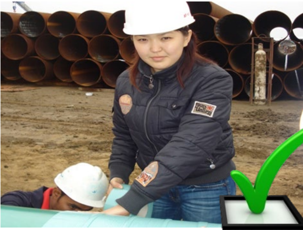
Apply Wrappingband without tension.
