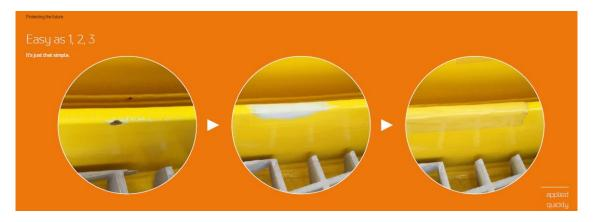
The unlimited shelf life of these products mean they can be used as and when any coating damage takes place either onshore or offshore. They are readily available in the standard colours (Grey RAL 7035 and Yellow RAL1023). EasyQote® SC Patch system can offer a cost-effective solution to corrosion that is designed to outlive the life of the asset itself.
