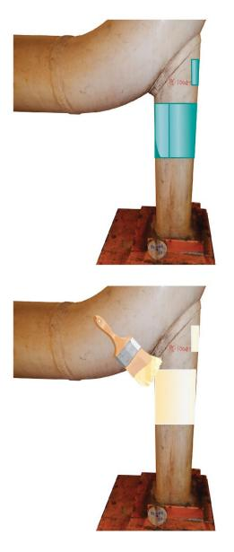
Apply EZ Wrappingband to secure the paste plug in place with a minimum 50mm adhesion to the substrate around the perimeter of the hole.
