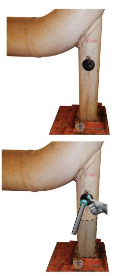
Clean and remove any loose debris from inside the trunnion where possible.
